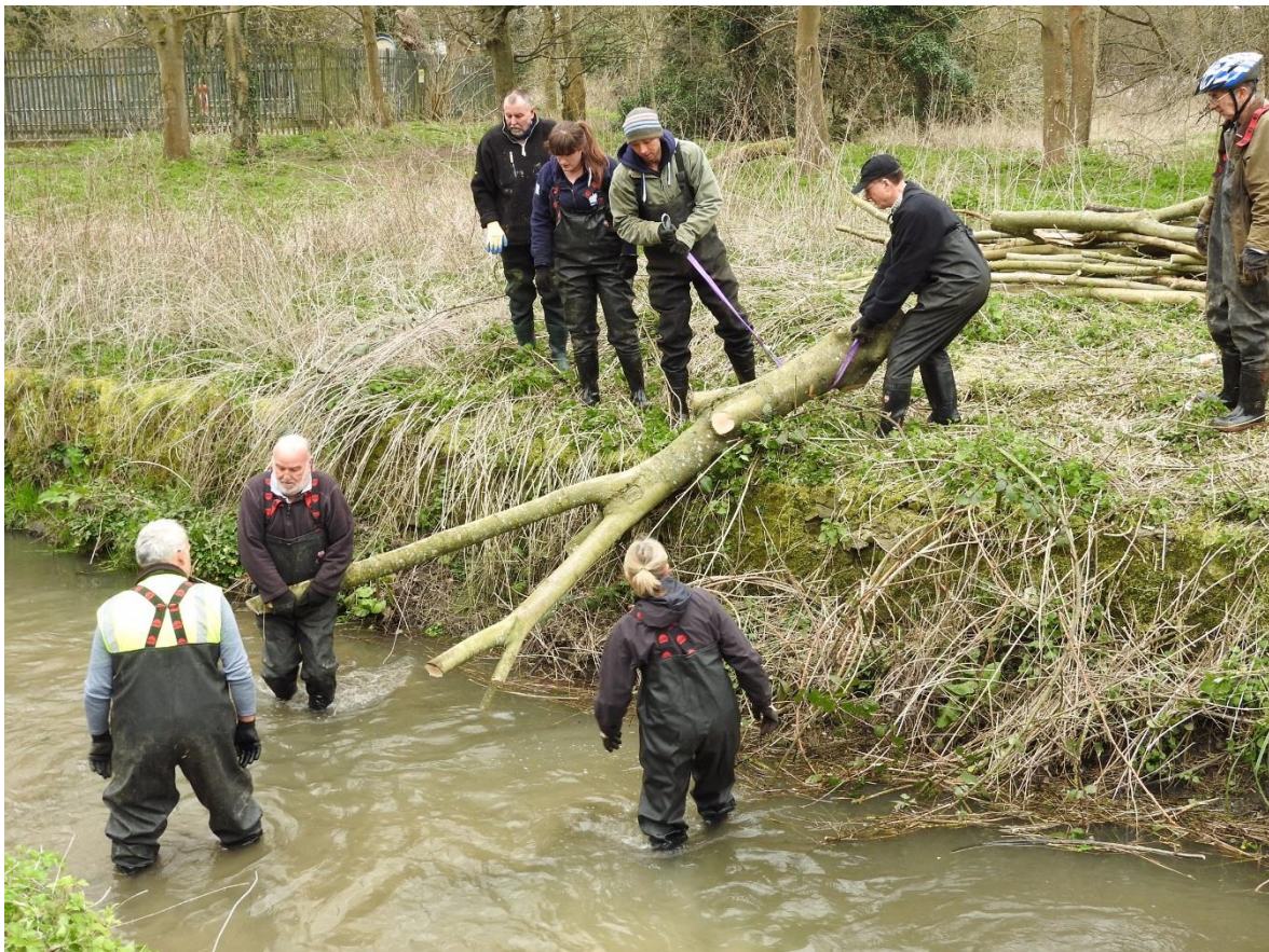
Hogsmill LNR, South East Rivers Trust staff and volunteers installing in channel features to improve the rivers habitats for fish
