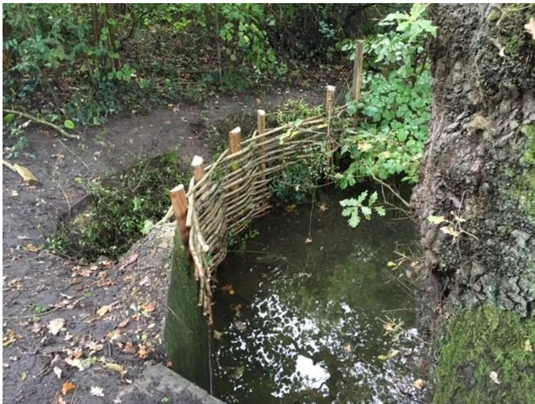
EEBC Countryside Team volunteers October 2020 completed repair of erosion caused by dogs on the banks of the Green Man Stream in Pond Wood on Horton Country Park LNR
